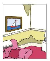
Rising damp will only affect basements and ground floor rooms. It will normally rise no more than 12 to 24 inches above ground level (300mm to 600mm) and usually leaves a 'tide mark' low down on the wall. You may also notice white salts on the affected areas.
